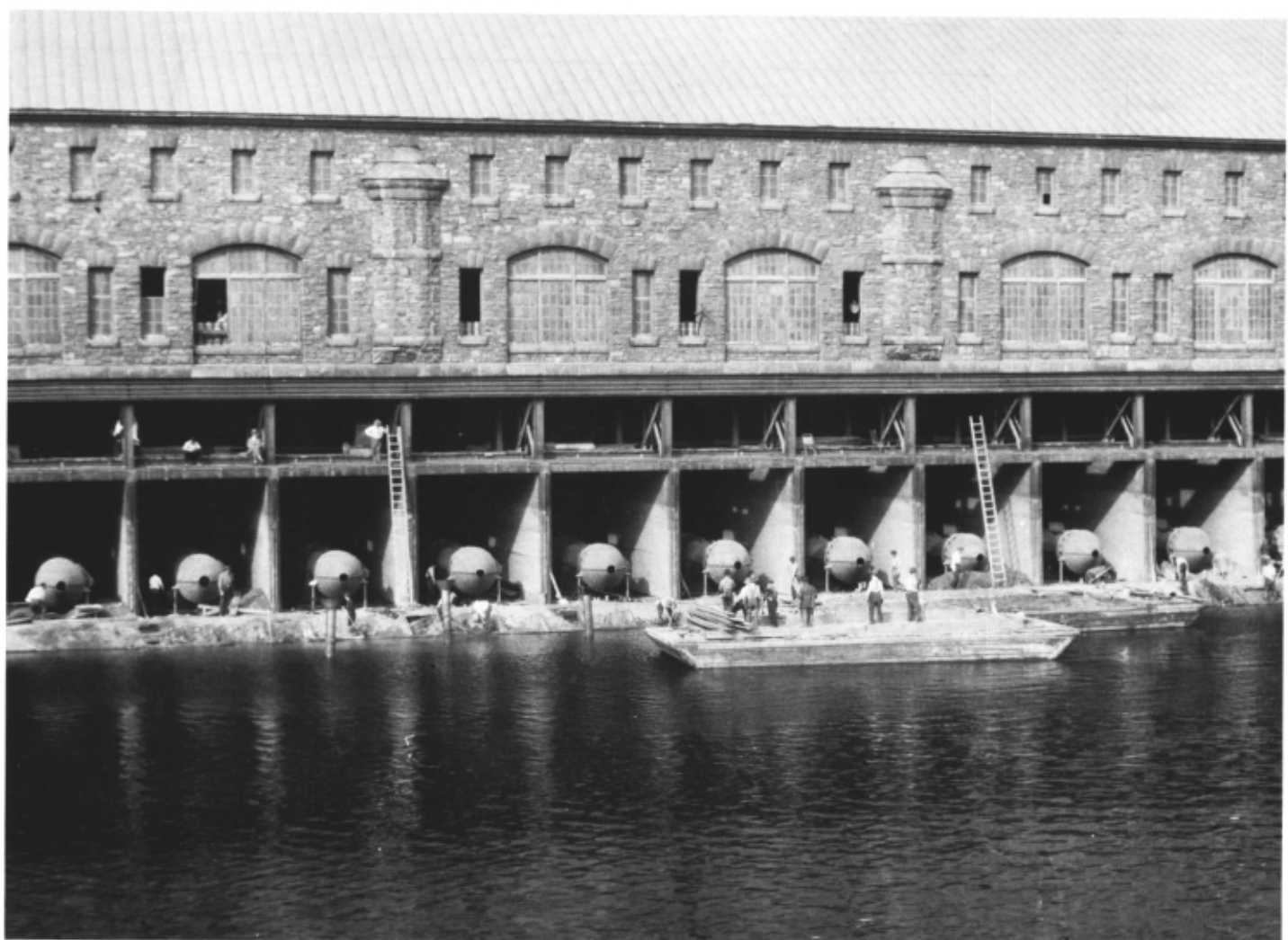
Forebay side of hydro plant during installation and construction of the turbines in 1902.
