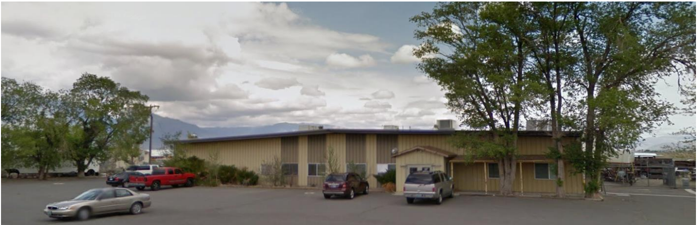
Location of original Bently Nevada Corporation building (rebuilt after the fire on Sunday, April 11, 1976). 1132 Airport Road, Minden, NV 89423.
